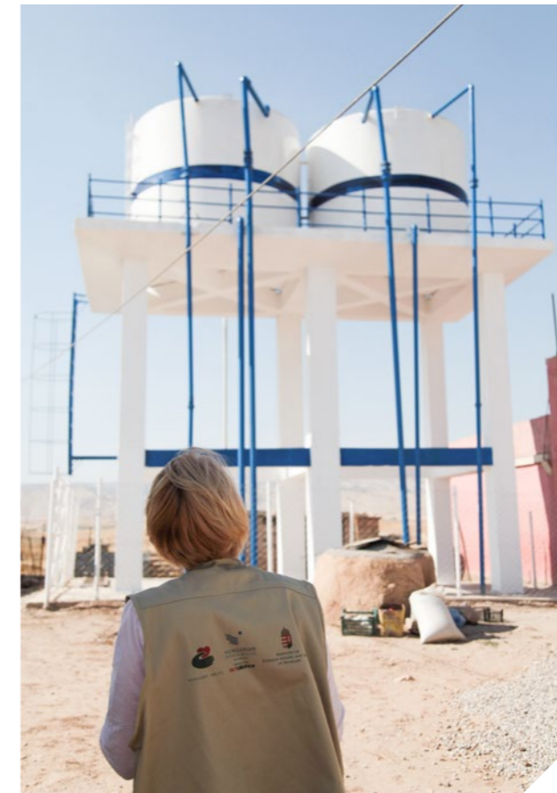
Water tank contributing to the local water supply in Iraq Source: Hungarian Interchurch Aid
